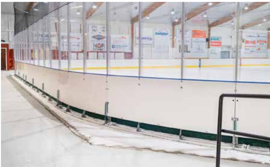
Installation into ice with steel plates
